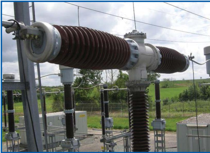
2. Two breaks per phase circuit breaker connected to ground on both sides
